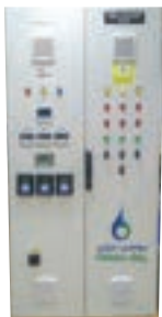
VFD Control Panel
