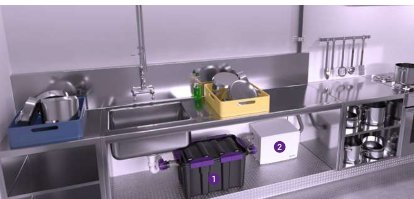
1 Grease separators 2 Lifting station
