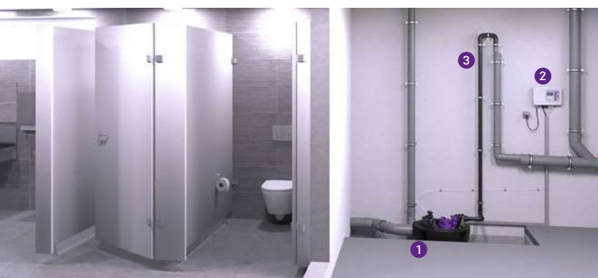
1 Lifting station 2 Control unit 3 Pressure pipe
