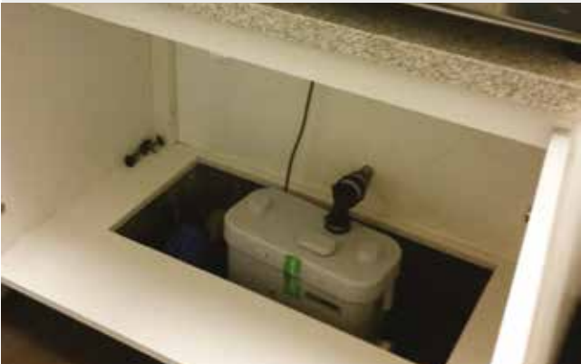
SANISPEED ® pump installed to remove kitchen waste water.
