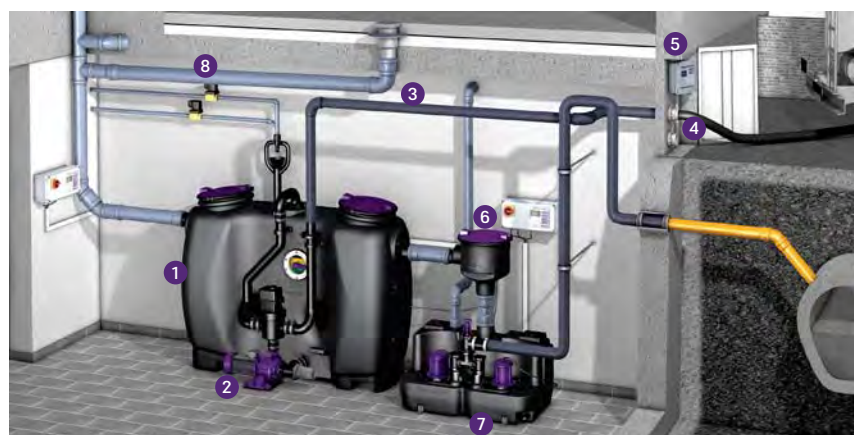
1 Grease separator 2 Shredder-Mix-System 3 Disposal line 4 Connection for disposal truck 5 Remote control system (optional) 6 Sampling chamber 7 Lifting station 8 Solenoid valves
