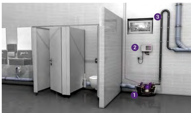
1 Lifting station 2 Control unit 3 Pressure pipe
