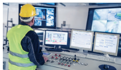
Remote Control Room
