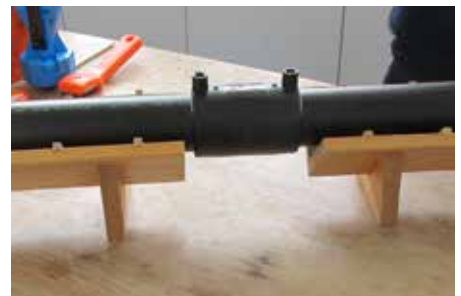
Electro weld process
