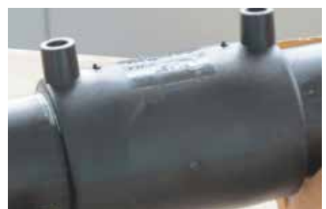
Finished electro fusion weld
