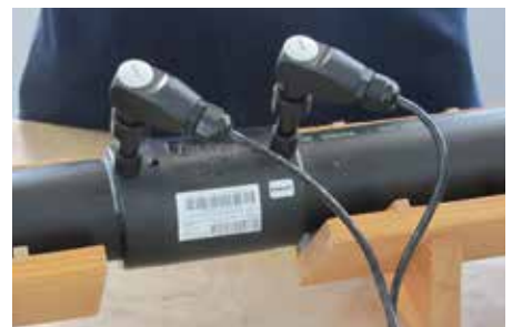
Finished electro fusion weld
