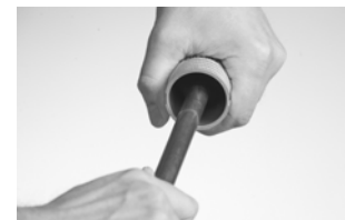
DEBURRING THE TUBE
