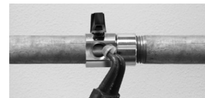
Remove the filter with pliers then clean or replace it
