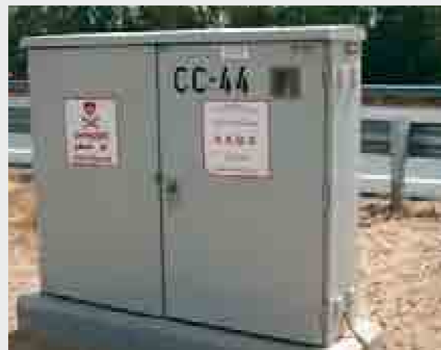
Street Lighting Cabinets at Dubai Silicon Oasis
