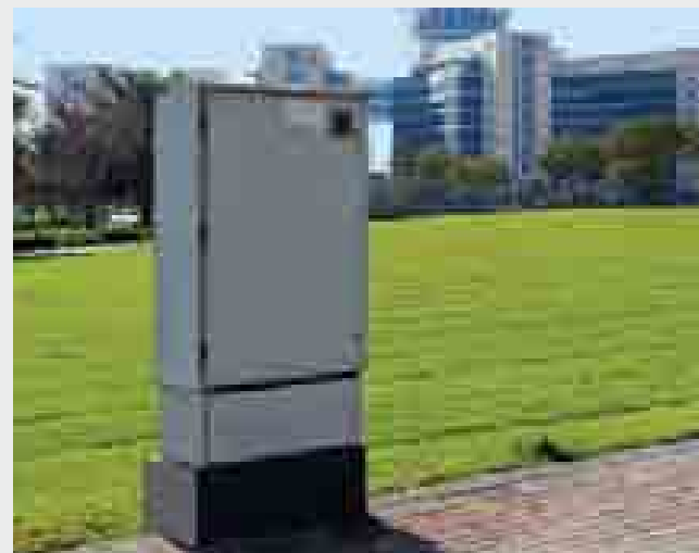
Street Lighting Cabinets at Dubai Silicon Oasis
