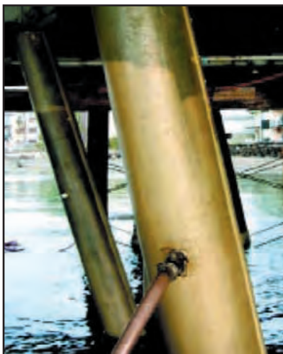
Pumping the 550 Grout. Note the visible rising level seen through the Form.
