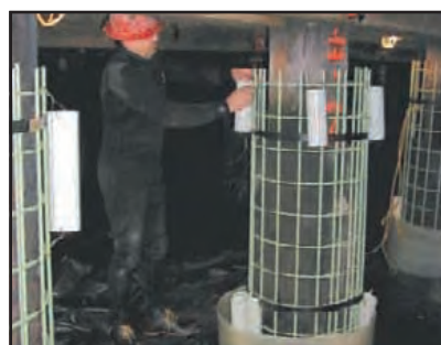
Placing the standoffs around the steel rebars before fitting the Fiber-Forms.
