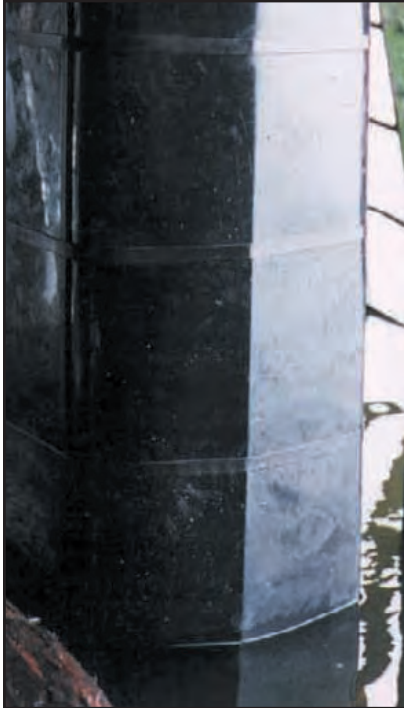
Hexagonal pile protected with SeaShield Series 100 system.
