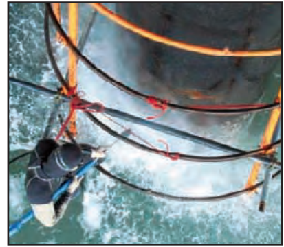
Cleaning using a high pressure water jet
