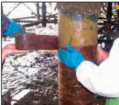
Applying Denso Marine Piling Tape.
