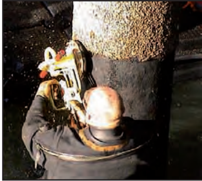
Cleaning with a power tool.
