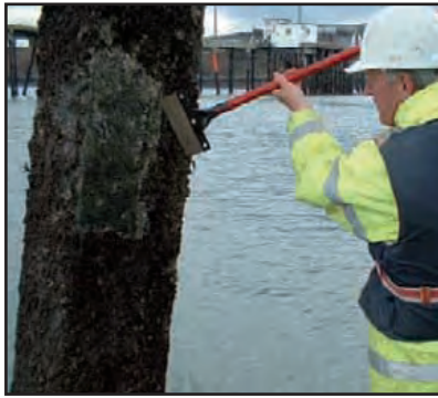
Cleaning with a hand scraper.
