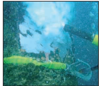
High pressure water jet under water.
