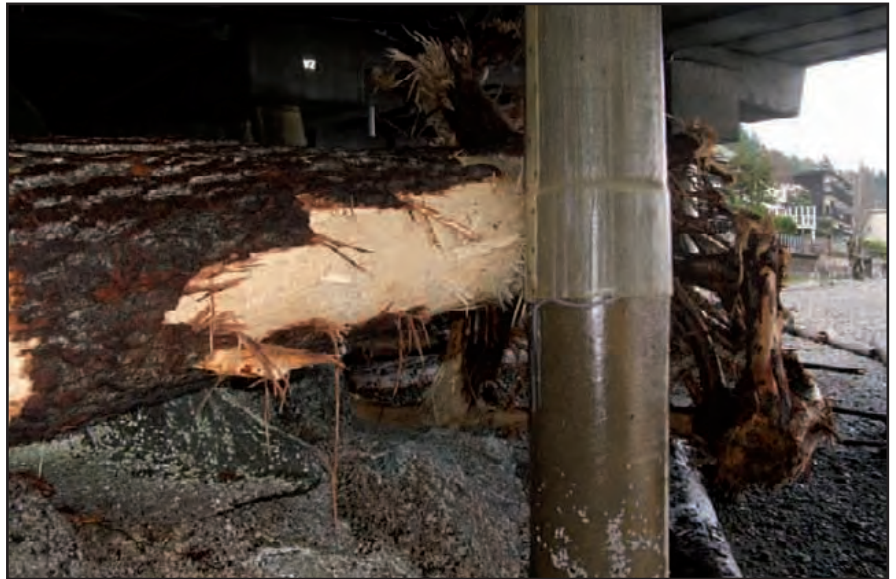
SeaShield 500 system still intact after withstanding a severe battering from this uprooted tree during a storm in the USA.
