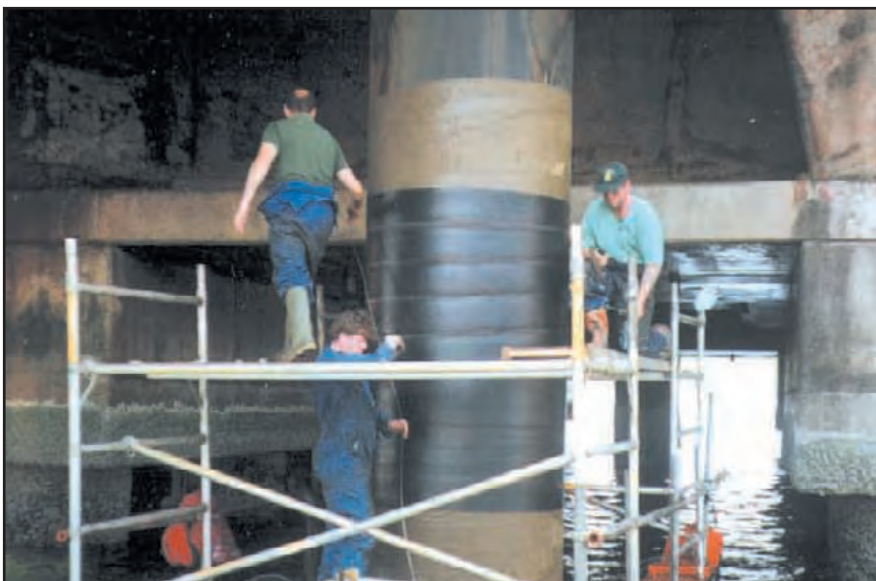
Installing the SeaShield 100 Jackets over the Petrolatum Inner Layer.
