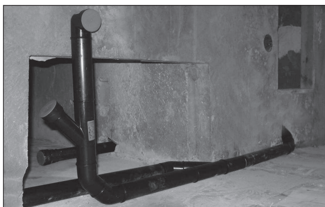
Illustration 9.2 Prefabricated pipe sections installed on site
